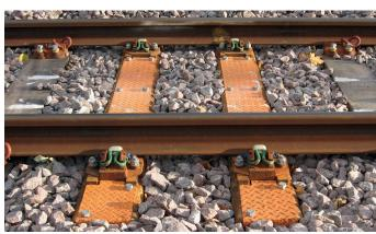
Our Hollow Sleepers are manufactured in the UK by Trackwork Ltd, with a fully comprehensive range covering all UK track configurations and easily adapted to suit all other major track systems.
